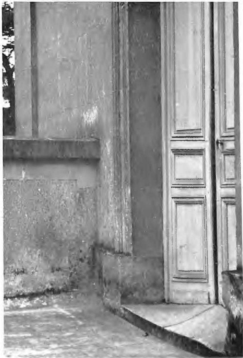
18. Detail of the Chapel Doors and Terrace Pre-coved stone flags turning the corner of the Chapel perron , upon which the walls are set. Mique may have cut through here to commence a communicating way to the maison (see Plate 19).
